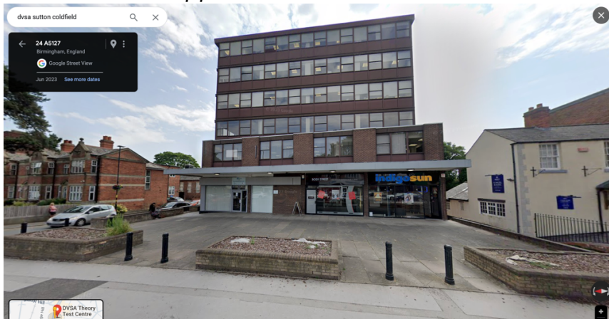
1X New litter bin approved for the front of the DVSA offices on Birmingham Road
